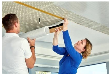
Align Cleaneo SYSTEXX Silent to the silicone tape.
